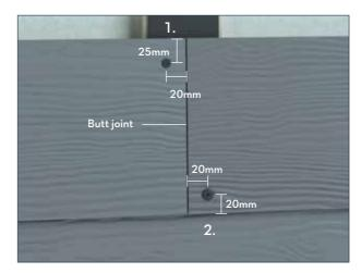
When butt jointing, make sure planks are loosely butt jointed.
