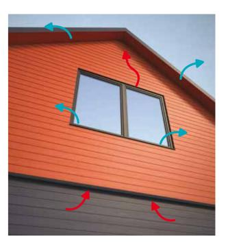
This passage must be a minimum of 10mm in the top and bottom or equal 100mm per m<sup>2</sup>. If grids or similar are used, the openings must equal 100cm<sup>2</sup> per linear meter.
