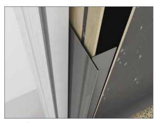
**NOTE!** If using unpainted aluminium in connection with fibre cement products, be aware of surface oxidation.
